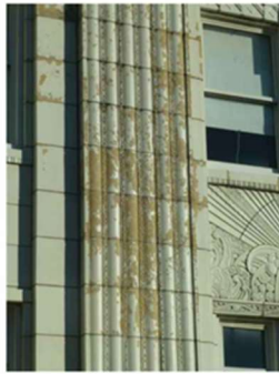
EXTENSIVE GLAZE SPALLING
