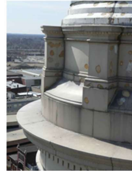
SIMILAR SPALLING ON ALLEN COUNTY COURTHOUSE
