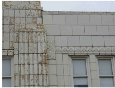
SPALLING DEPENDENT ON FABRICATION RUN AND EXPOSURE
