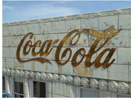
SPALLING OCCURS IN BOTH WHITE AND GOLD GLAZES
