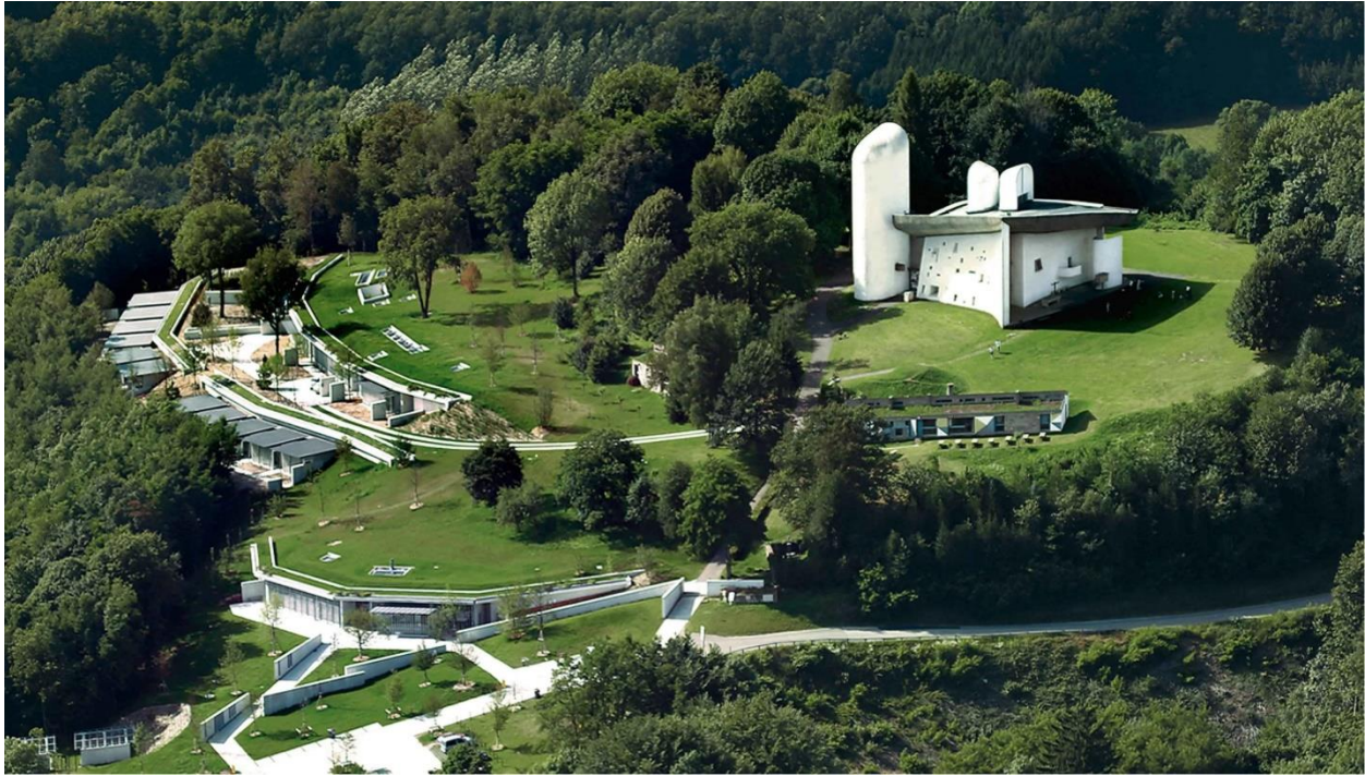
Figure 7: Rochamp complex including gatehouse, monasteries and chapel. https://arquitecturaviva.com/works/acceso-y-monasterio-10
