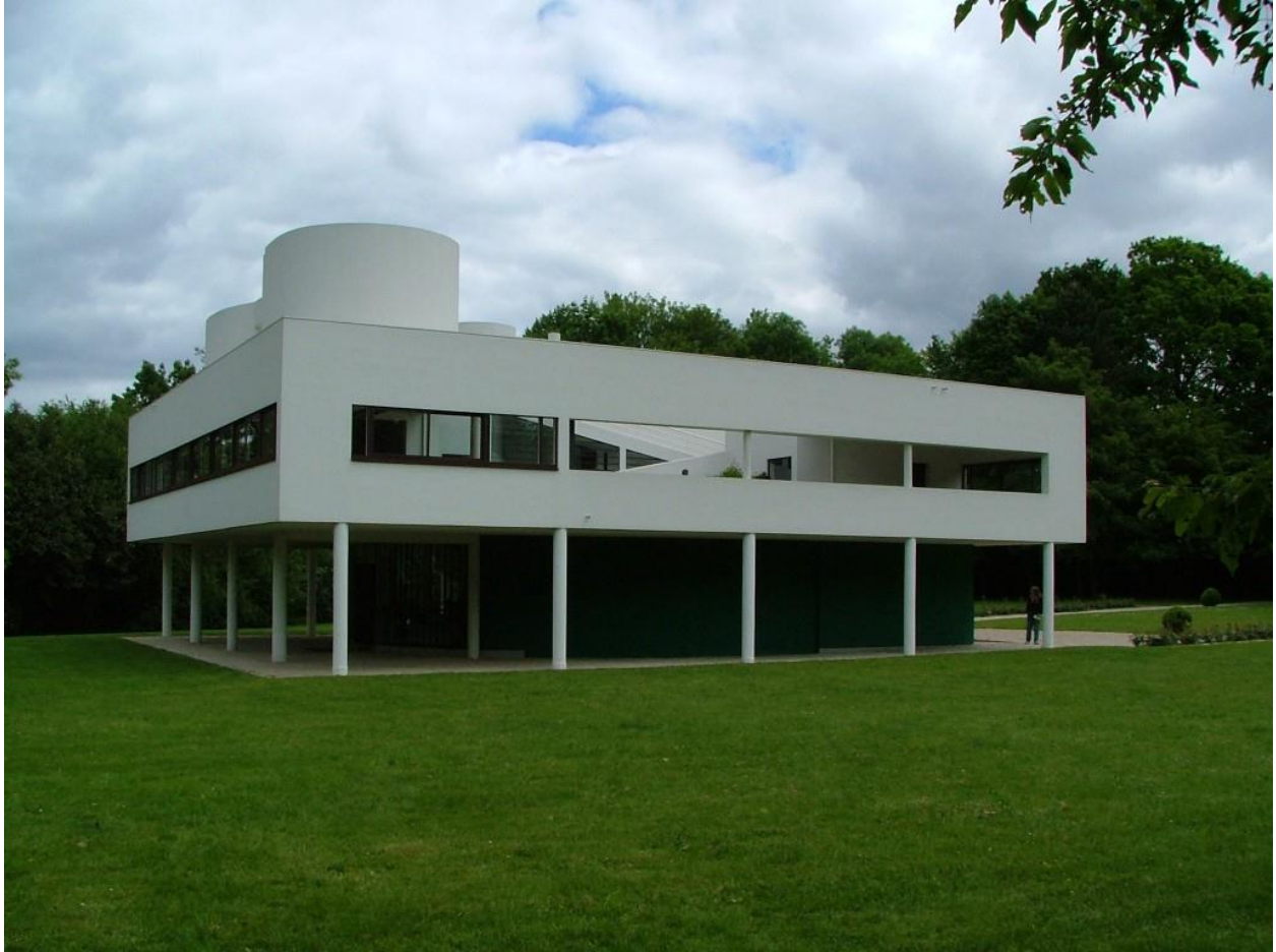
Figure 12: Le Corbusier, French, Swiss, architect. 1929-1931, Image: Saturday May 22, 2004 -- 01:29:01 PM. Villa Savoye. Residential Buildings. https://library.artstor.org/asset/ASAHARAIG_1113118960 .
