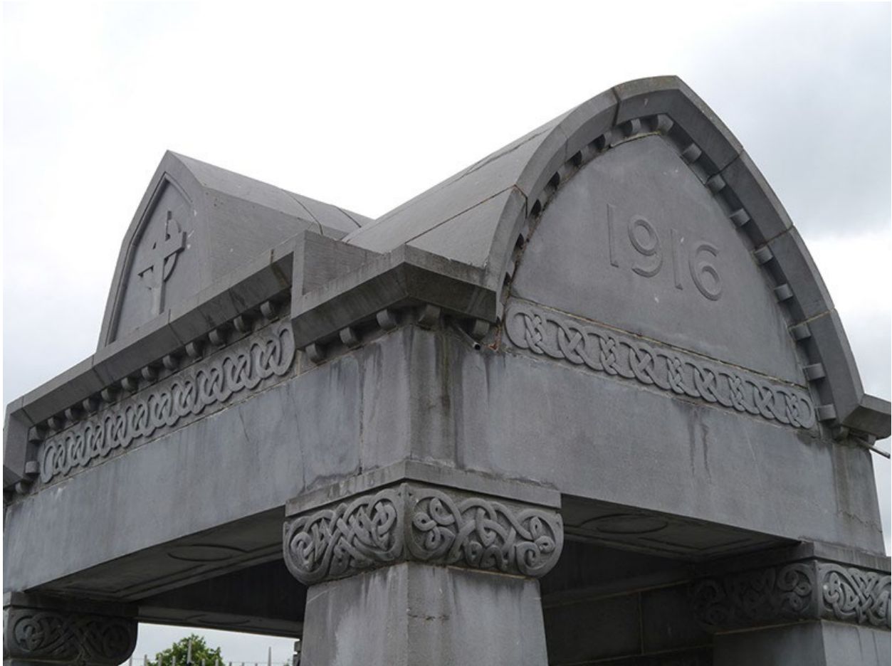
Figure 4. Dora Sigerson Shorter. Sigerson Memorial (Detail of Gables)- A monument to Pádraic Pearse and his comrades, shot in Easter week. 1918 (monument complex completed 1927). Carrera Marble in an Ashlar Limestone Pergola. Glasnevin Cemetary, Dublin, Ireland.
