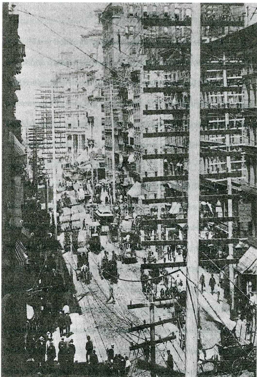
Fig. 4 "New York street scene—before wires were placed in cables beneath the streets" (Todd 35).
