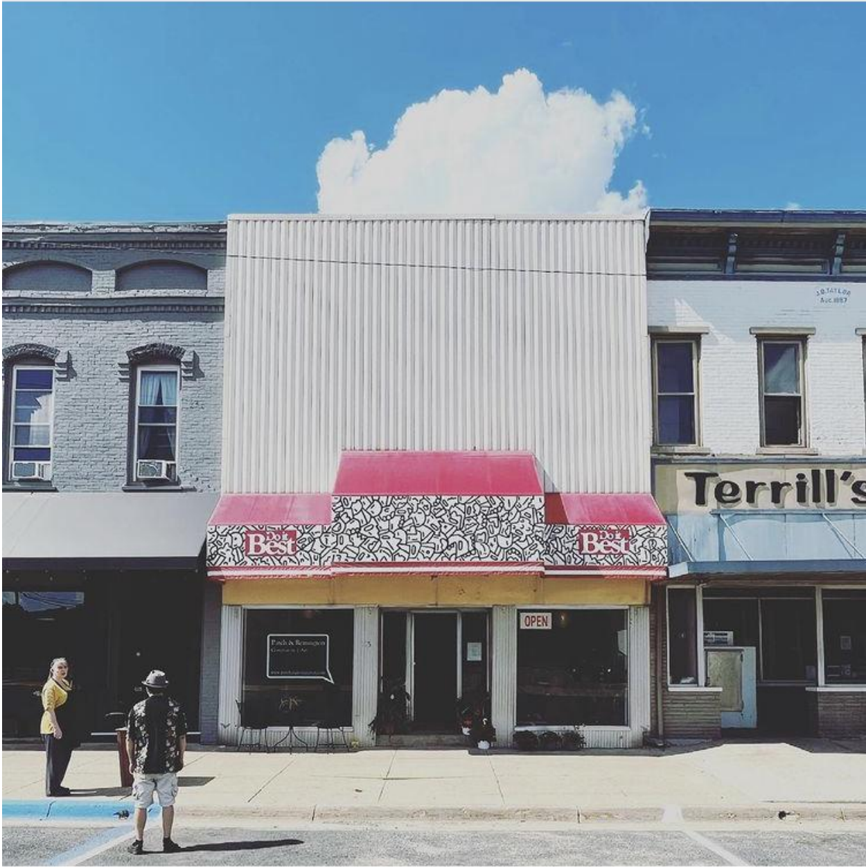
Figure 6, Patch & Remington, Courtesy of Mike Han, photograph.
