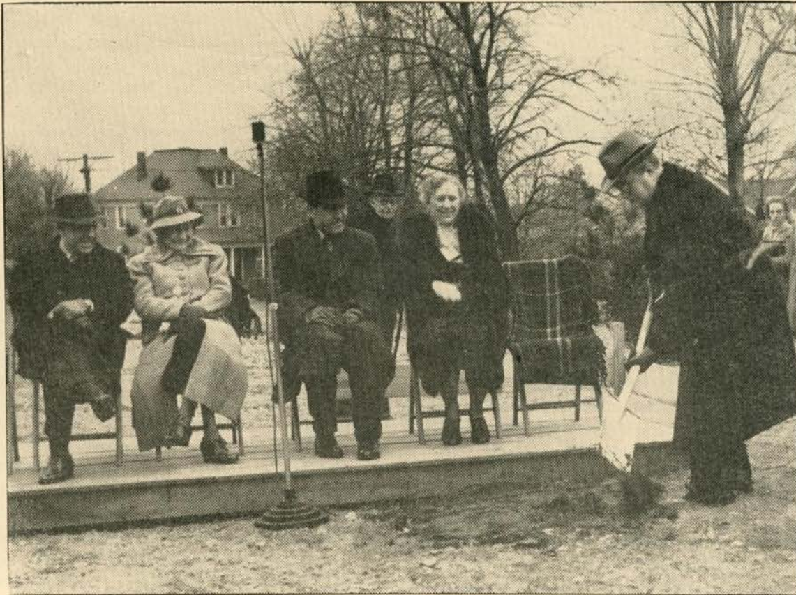
Breaking Ground for the Lillie P. Roemer Memorial Fine Arts Building, February 14, 1939.
