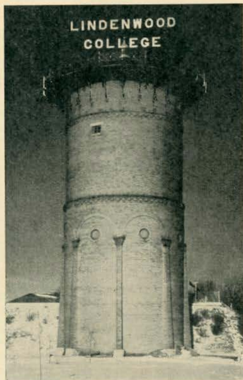
The Water Tower, with its Lindenwood sign blazing by night in bright red neon letters, has long been a landmark to motorists along U. S. Highway No. 40, and to students returning to Lindenwood. It was one of the many improvements made on the campus during Dr. Roemer's administration.
