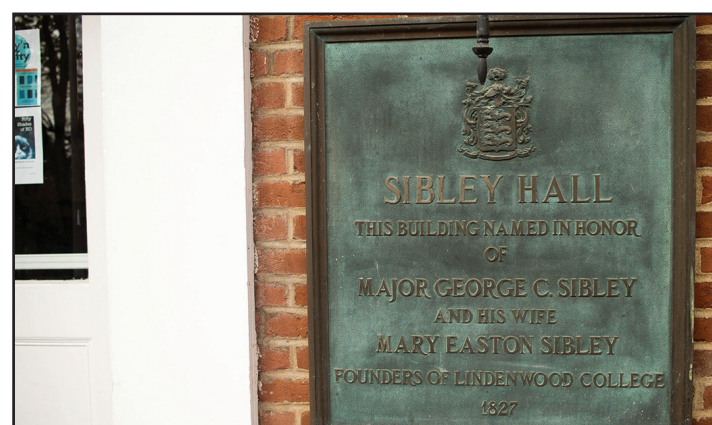
Photo by Kelby Lorenz Sibley Hall is the oldest dorm on St. Charles campus, and due to a roof issue, students have now been forced to move out.
