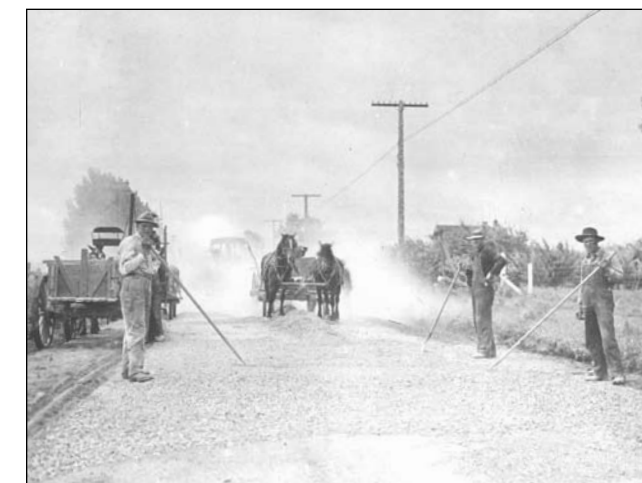
Macadam roads were still being built in the twentieth century, as seen in this photo from Oregon. (Photo: Oregon Department of Transportation, History Center)
