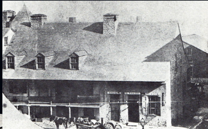
Robidoux House, front (top) and back (bottom), bakehouse in the rear (with pointed roof), photographs by Thomas Easterly. (Images: Missouri Historical Society, St. Louis)
