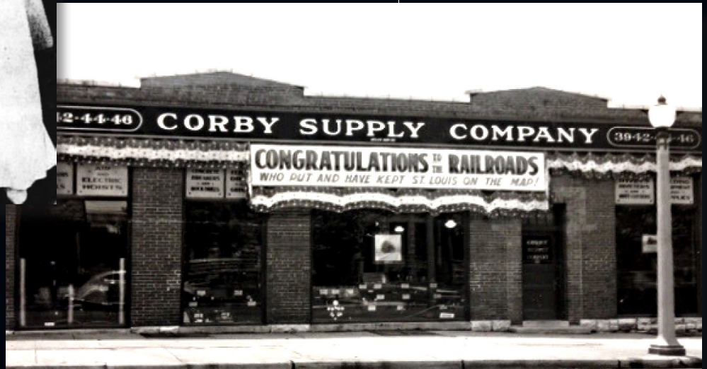
Corby Supply Company Headquarters in St. Louis, Missouri. (Image: Stephen L. Kling, Jr.)
