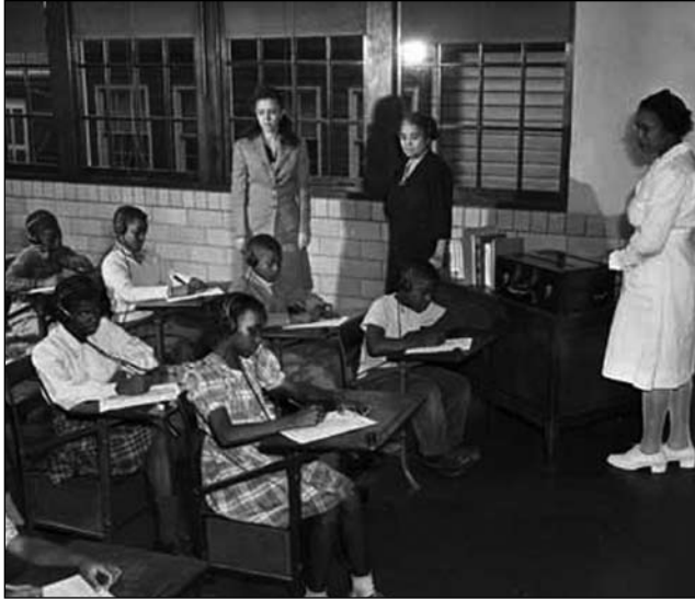
J. Milton Turner School, pictured here, was the most prominent public building in the Meacham Park community (later annexed by the City of Kirkwood). Meacham Park was a predominantly African American neighborhood in St. Louis County; in 1925, Kirkwood Public Schools completed Meacham Park School to replace the aged and substandard Booker T. Washington School. It was renamed J. Milton Turner School in 1932, commemorating James Milton Turner (1840-1915), a former slave who became a prominent politician after the Civil War. (Photo: Western Historical Manuscript Collection, St. Louis)
