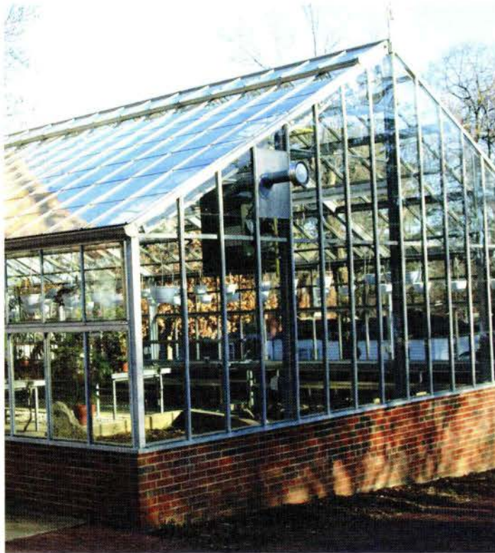
The Monsanto Greenhouse at Young Science Hall was completely renovated in 2006.
