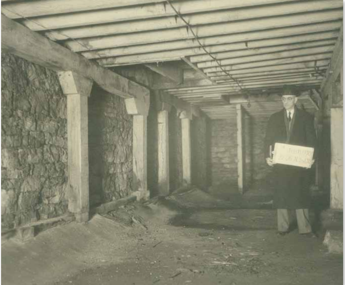
The basement at 22-26 North Second Street. Before structural steel, a three-story building required a wide stone foundation and massive wooden beams. (Image: National Park Service, Jefferson National Expansion Memorial Archives, Record Unit 106.8-5 Parcel Files)
