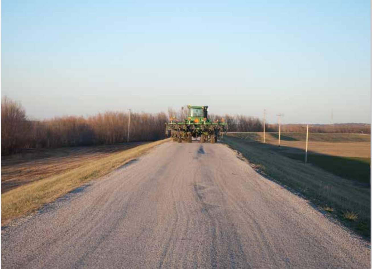
Levee Road near Fountain Creek
