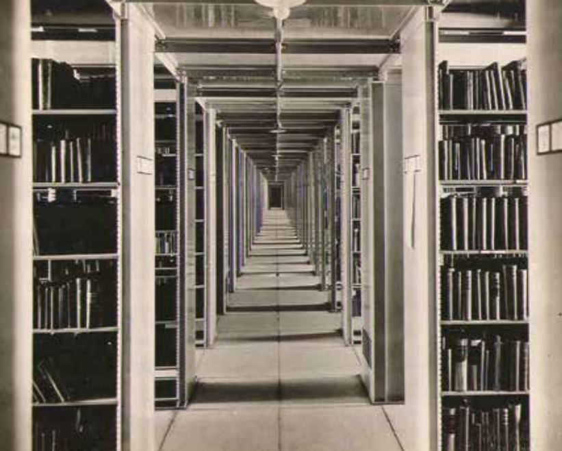
Stack tower, 1912. F.D. Hampson Commercial Photographer.
