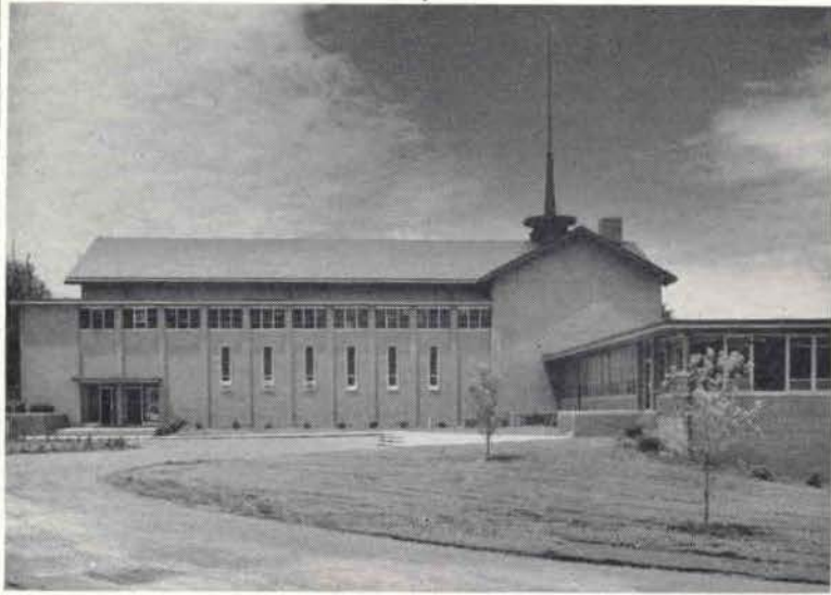
Exterior of the finished chapel
