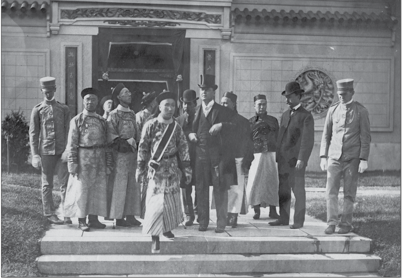
After the initial reception, Prince Pulun and Fair President Francis tour the Chinese contribution to the exposition, including the Chinese pavilion. The latter was constructed to resemble a palace belonging to Pulun in northern China. (Image: Missouri History Museum)
