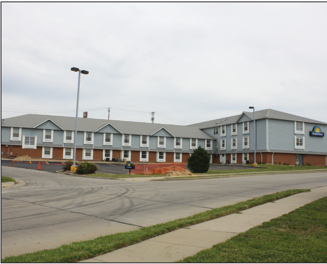
The former Days Inn motel (left) located on Veterans Memorial Parkway is now the "Linden Lodge." The Lodge is now the largest residence hall, housing about 200 men. Areas in the motel like the breakfast room (top right) and main lobby remain for student use. Most rooms (bottom right) in the Lodge are two person occupancy, featuring the same amenities as
