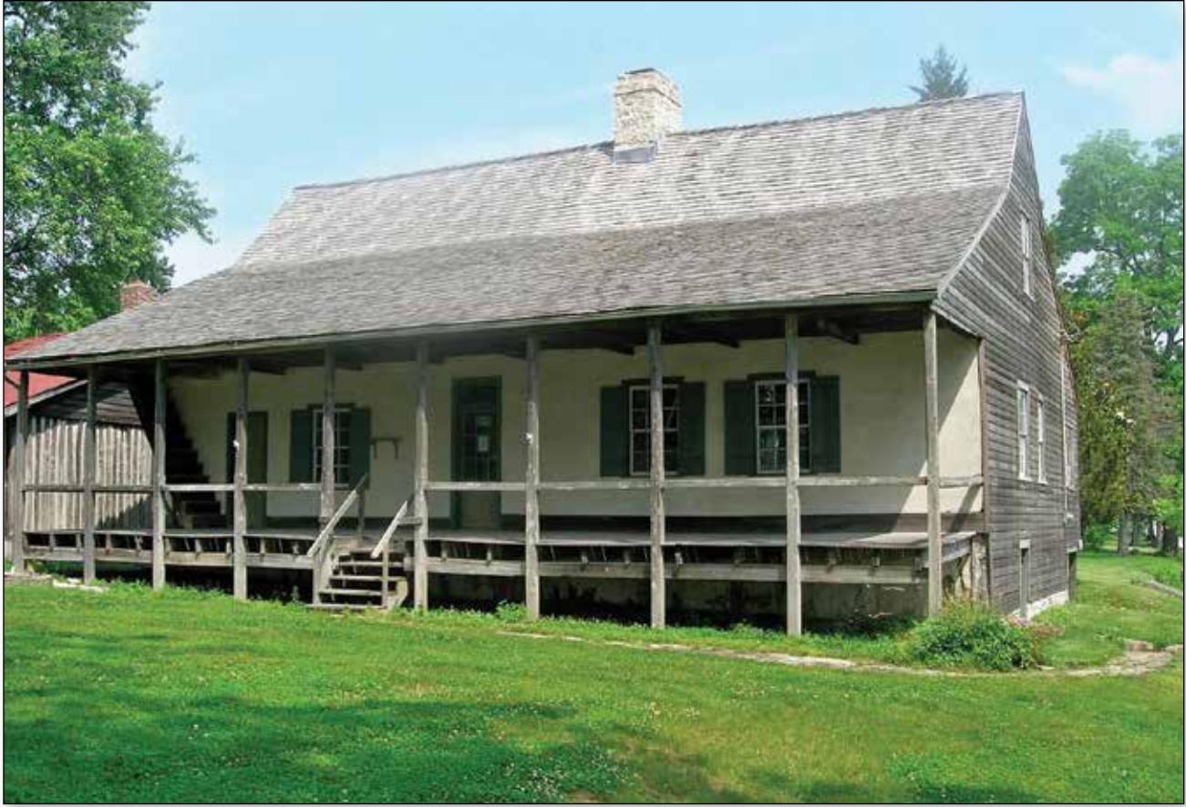
Amoureux House, 327 St. Mary Road, constructed c. 1792, was the home of Pelagie Amoureux in the mid-1800s. (Image: Courtesy of the Author)
