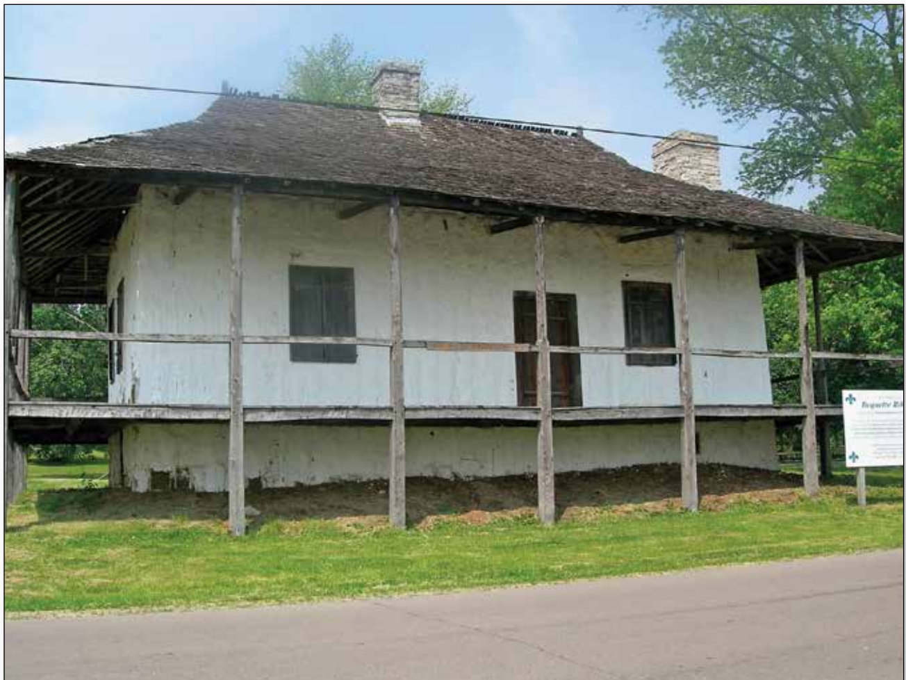
Bequette-Ribault House, 351 St. Mary Road, c. 1808, displays a galerie (gallery) all around. (Image: Courtesy of the Author)
