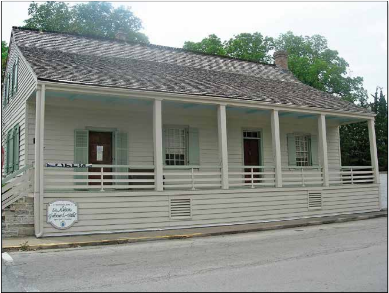
Guibourd-Valle House, 1 North Fourth Street, c. 1806, belonged to the Guibourd family, which was associated with Michel Badeau. (Image: Courtesy of the Author)
