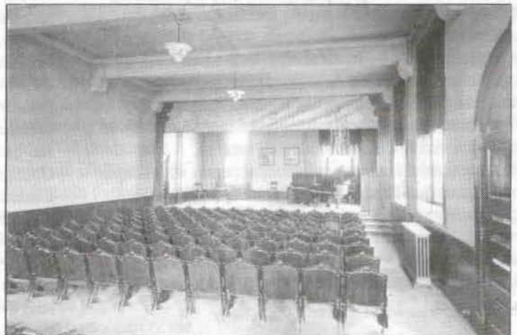
The chapel/assembly hall in Sibley Hall, as it appeared in 1907.
