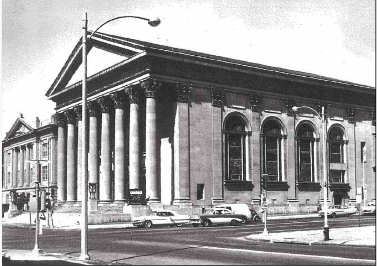
Temple Israel was among the religious institutions at the “Holy Corners” area in the Central West End at the intersection of Kingshighway and McPherson, and it was the synagogue for the large Jewish population in the West End. (Image: St. Louis Jewish Community Archives)
