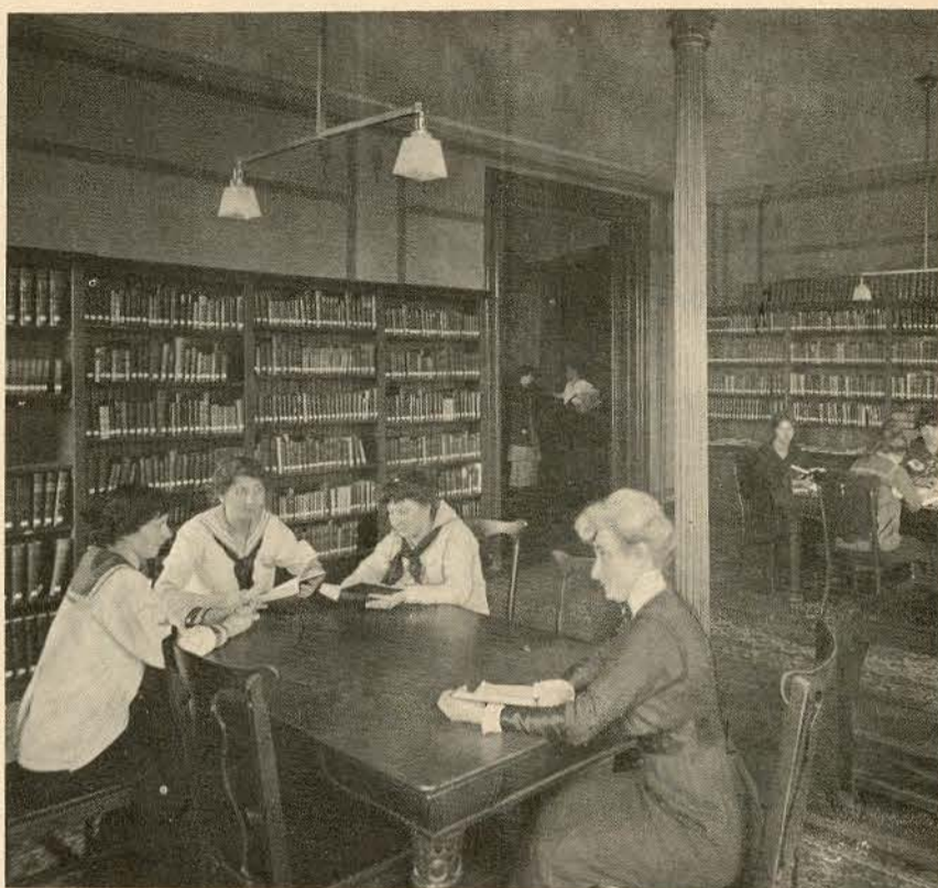
ELECTRIFYING —The new light fixtures add efficiency to the reserve shelves.
