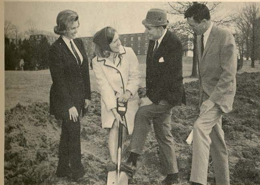
Ground Breaking —Mrs. Fern Bittner, Karen Mueller, Pres. John A. Brown, and Charles McGhee, designer-constructor, break ground for the new stables.
