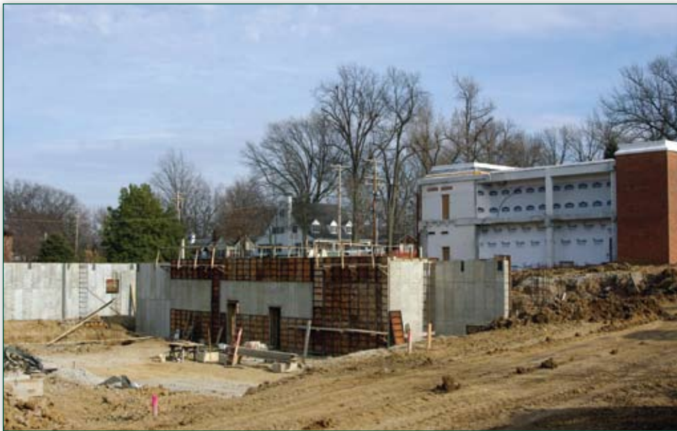
A major renovation to Harmon Hall is well under way.
