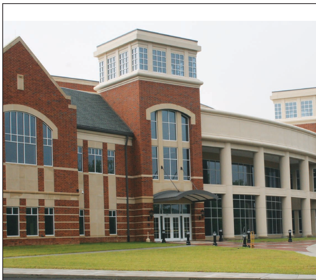
Legacy photo by Chelsea Lewis Although the completed exterior of Lindenwood's new Fine and Performing Arts Center looks serene, workers inside scramble to prepare the building's main stage for major headlining shows scheduled for this school year.
