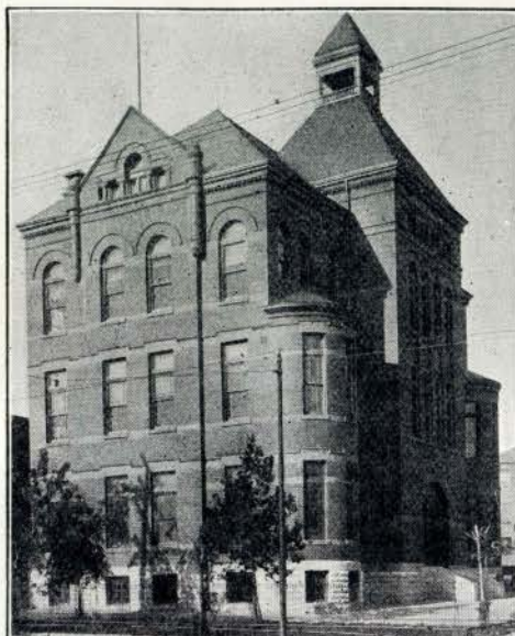
Jefferson Avenue Building
