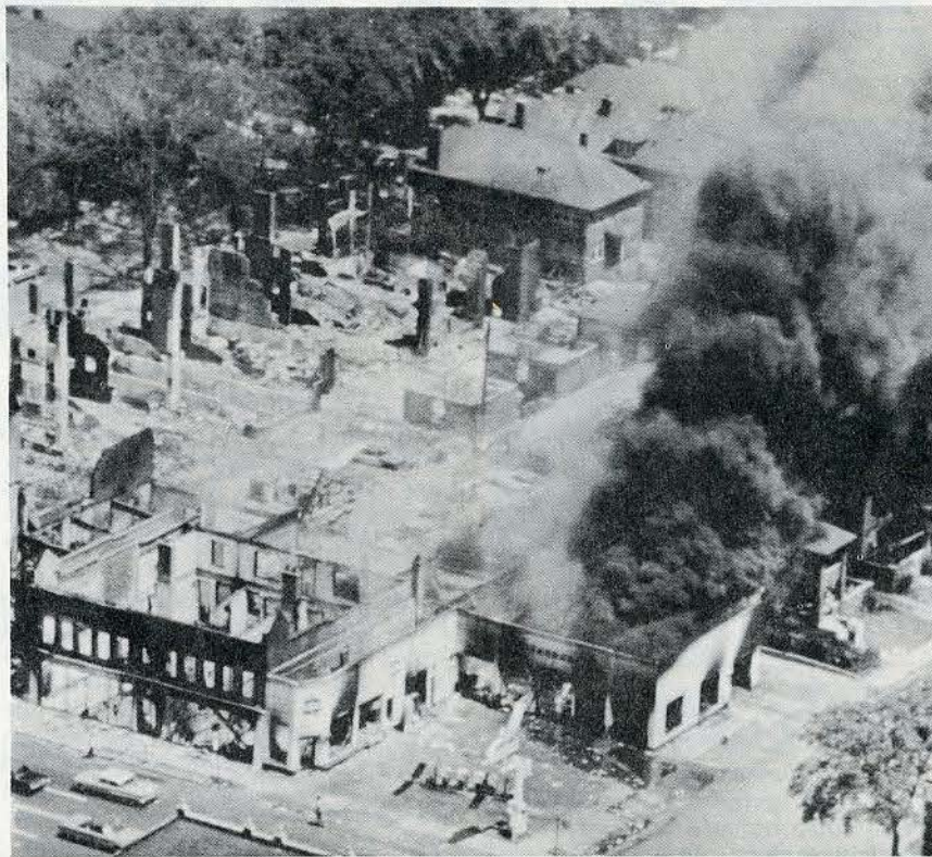
Detroit—The gutted remains of buildings (left) attest to the destruction caused by rioting in Detroit's West Side. A service station continues to burn (right) pouring smoke and flames into other structures.
