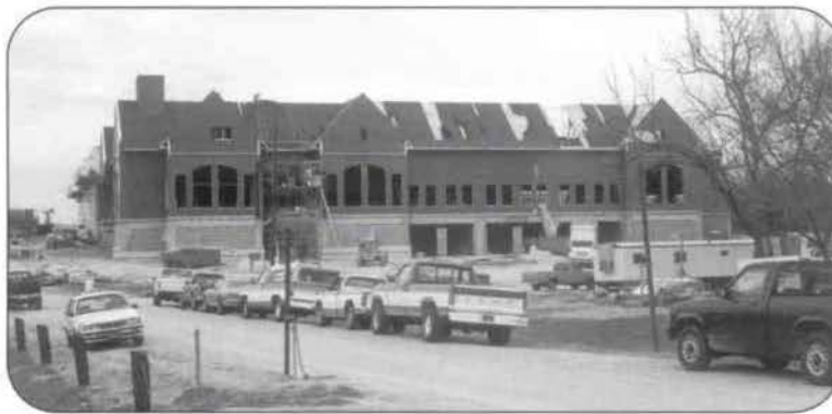
The Performance Arena takes shape.
