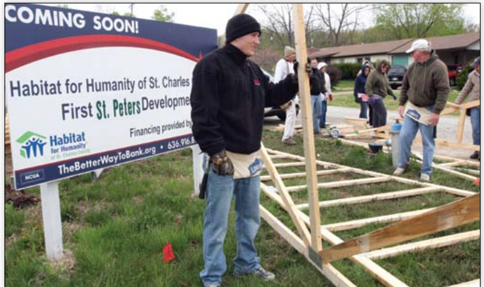
Jacob Johnson, education major, working on a Habitat for Humanity project.
