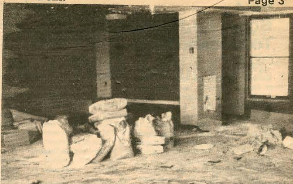
Student Center in Niccolls Hall near completion.
