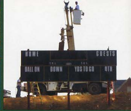
Construction workers finish installation of the new Hunter Stadium scoreboard
