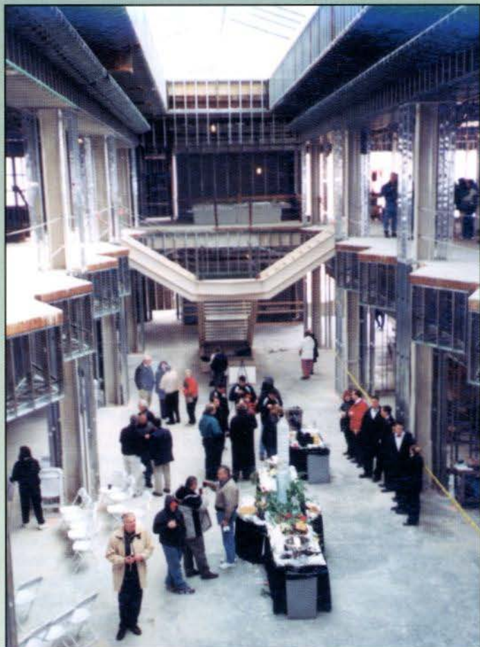
The Mabee Gallery Under Construction.
