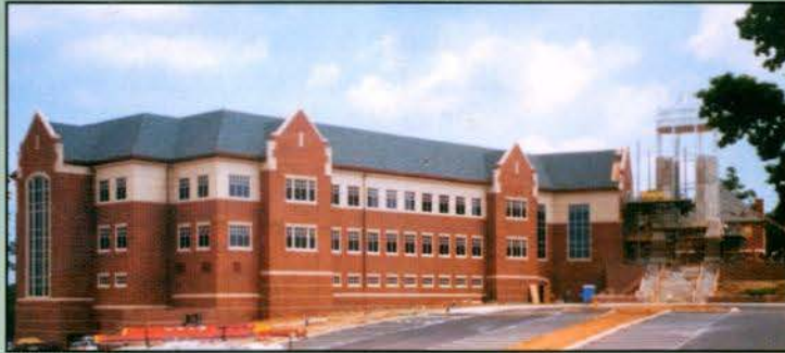
The Spellmann Campus Center gets some finishing touches as it prepares to greet students in 2002.
