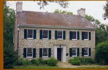
The historic Daniel Boone Home underwent substantial renovation in 2005.
