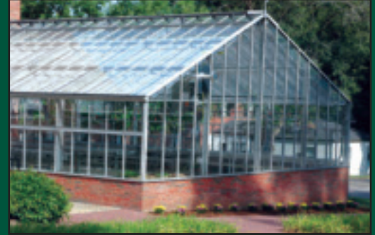
Renovations are under way at the Lindenwood University greenhouse
