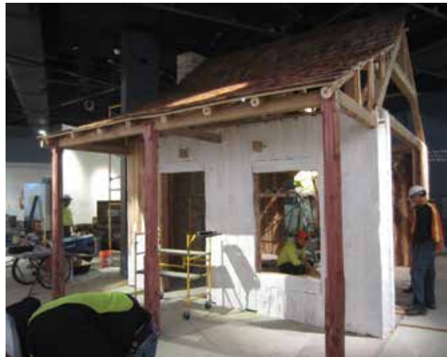
A 15 x 15-foot French vertical log house is the centerpiece of the Colonial St. Louis gallery, which describes the first 40 years of the city's existence and the changes brought by the Louisiana Purchase of 1803. The replica house, with two sides completed and the other two left unfinished to reveal building techniques, is the same size as several of the smallest homes in the early town. (Image: National Park Service, Gateway Arch National Park)
