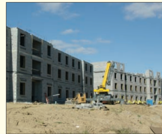
Two new residence halls under construction.
