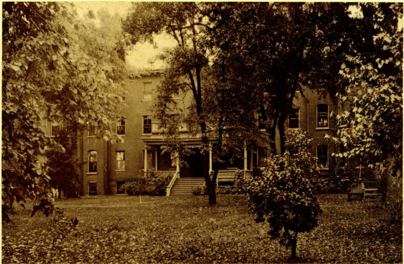
SIBLEY HALL—CLASSROOM, LIBRARY, INFIRMARY, CHAPEL, DORMITORY
