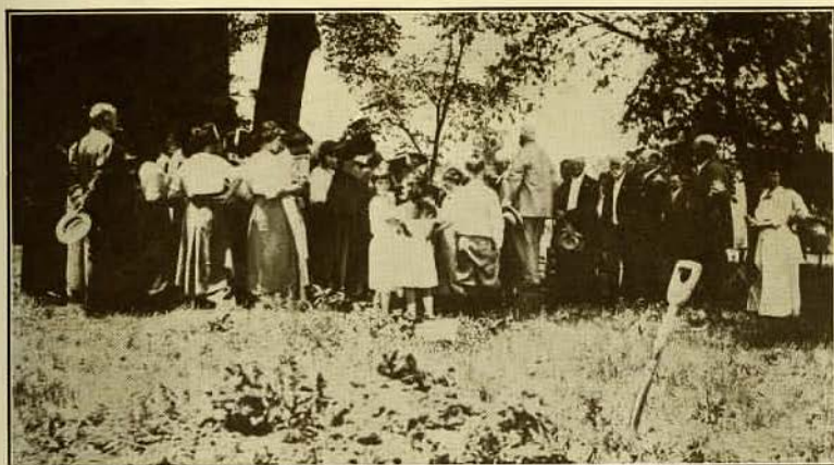
Breaking Ground for Butler Hall
