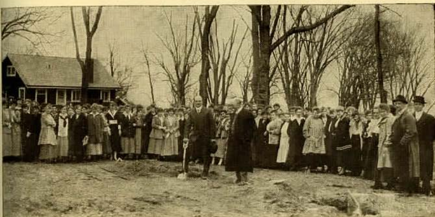
Breaking Ground for Nicolls Hall
