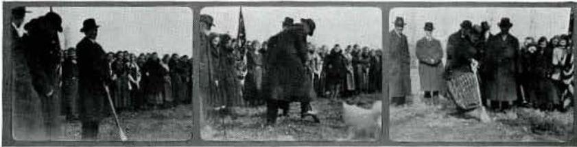
BREAKING GROUND FOR THE NEW ADMINISTRATION BUILDING FEBRUARY, 1920
