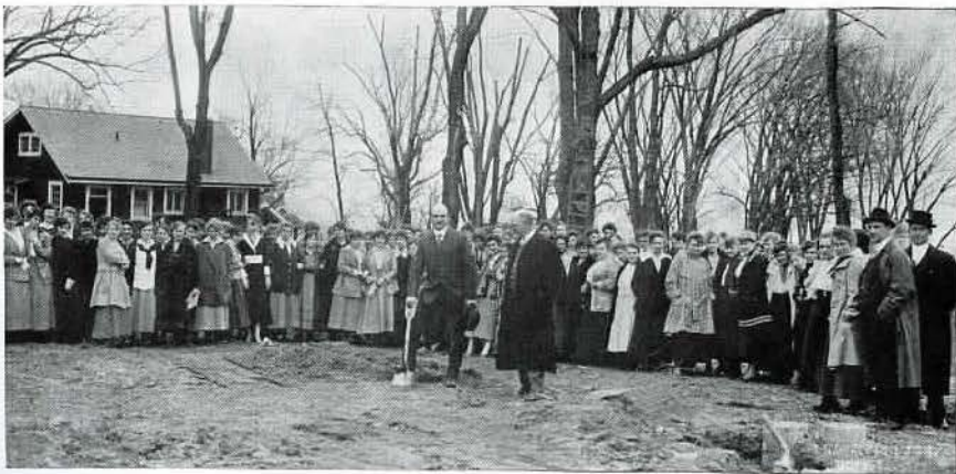
Breaking ground for Nicolls Hall.
