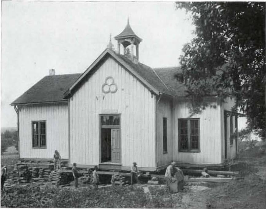
MOVING THE GYMNASIUM IN 1907 (SO THAT JUBILEE COULD BE BUILT)
