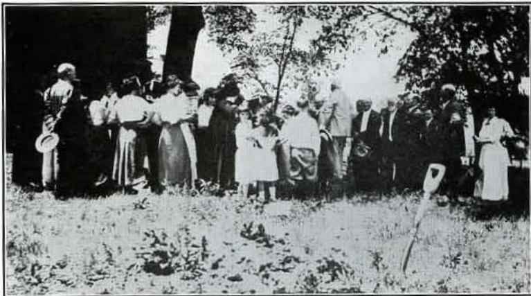
BREAKING GROUND FOR BUTLER HALL Col. Butler to right of center
