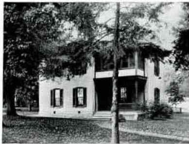
EASTLICK HALL (A Faculty House)
