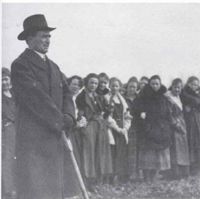
Ground was broken for Roemer Hall, built for classrooms and administrative offices, in 1920.
