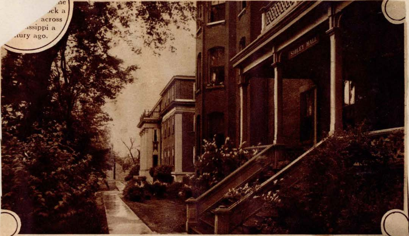
Sibley Hall at Lindenwood College, St. Charles. This, the oldest building on the campus, was named after Major George C. Sibley who founded the school in 1828.
